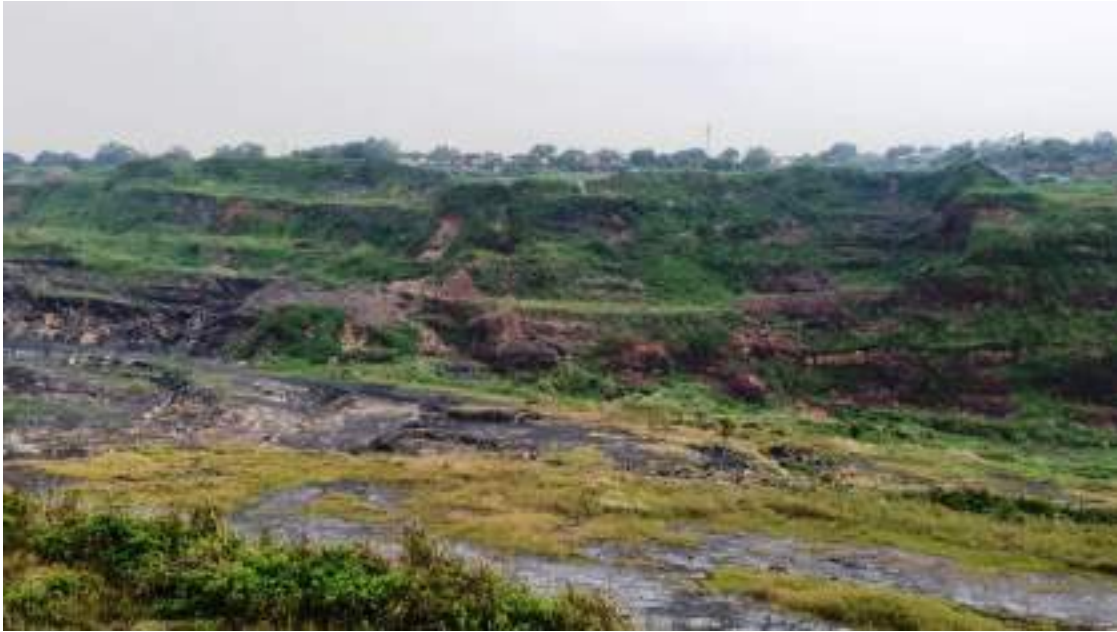
Figure 19: Subsidence area in Bagdigi Mines
