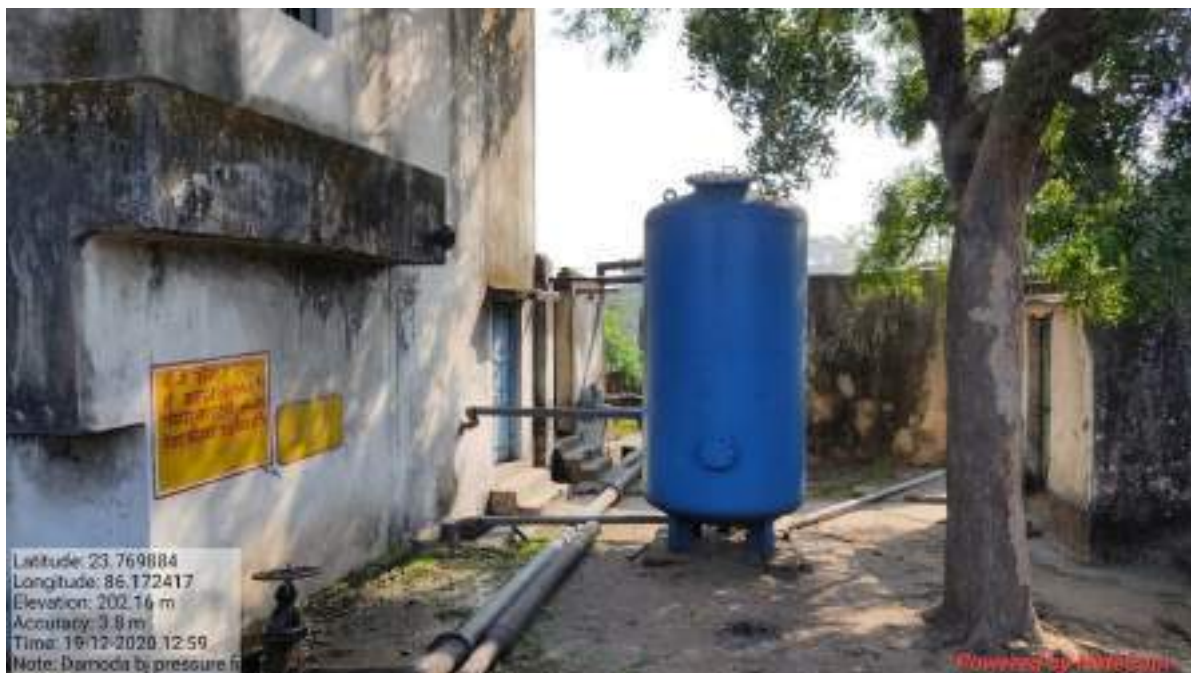
FILTER PLANT IN THE MINE AREA
