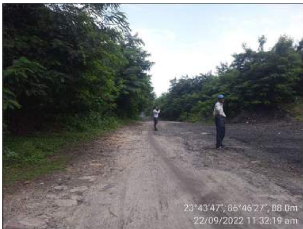
Photo 4: Plantation on Backfill in Cluster XVI
